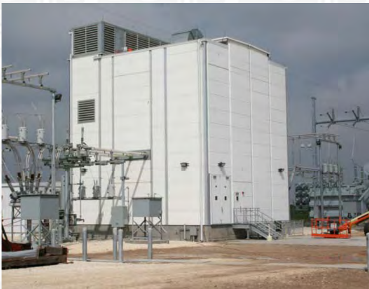
Variable Frequency Drive (VFD) Sound / Weather / Security Enclosure
