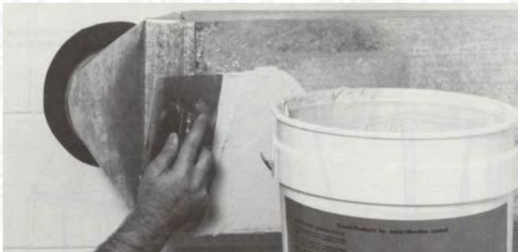
DC-10 applies easily to solid non-porous surfaces such as sheet metal with a trowel, brush, or airless sprayer.
