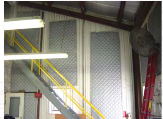
Custom Wall Blankets in a Seed Sorting Facility
